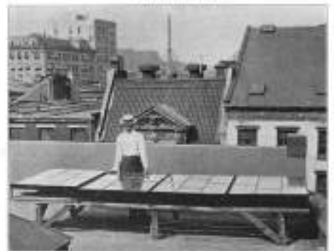
Mr. Cove and his solar electric dynamo. These solar heating panels are a feature of the house, and the man is standing by the apparatus which is the source of the solar energy.
